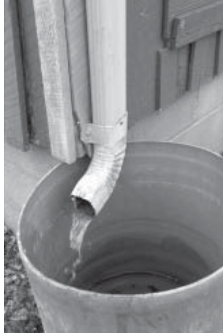
Suggested rain barrel design.
